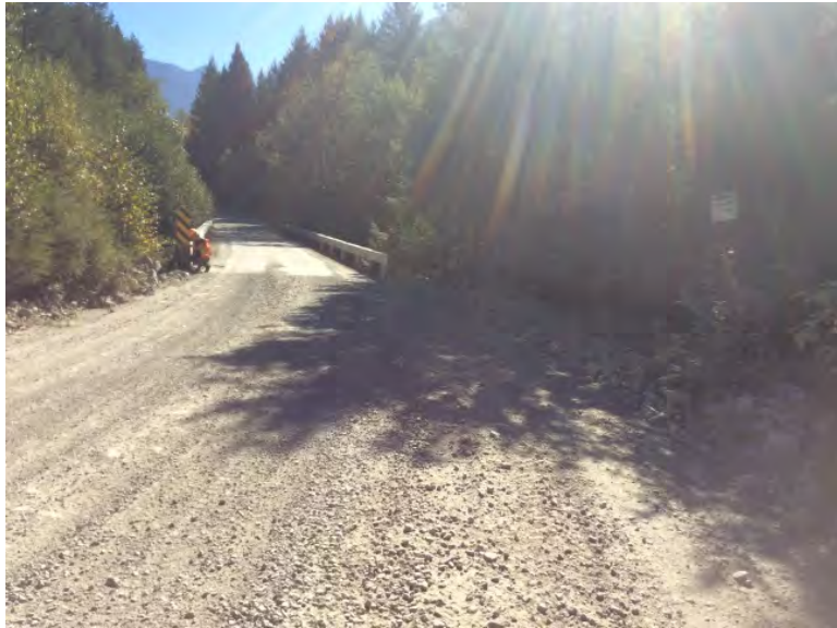
Approach from Left Bank when facing downstream
