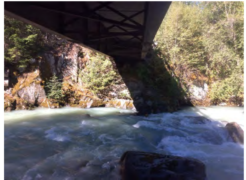
Left Bank Abutment when facing downstream
