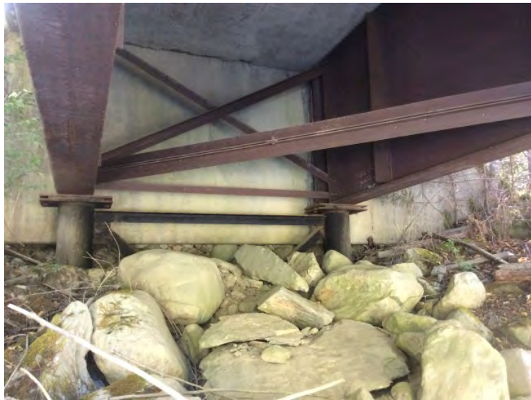
Right Bank Abutment when facing downstream
